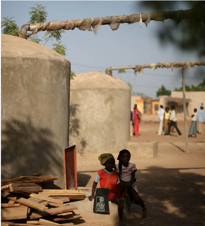
Rainwater harvesting tanks in Fana, west Mali, where water is scarce.
